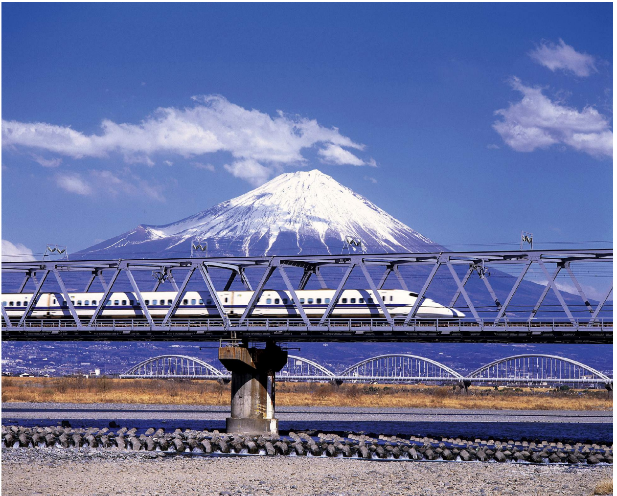
Fig. 10. The Japanese Shinkansen on its separated track, next to Mt. Fuji
